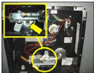
Water Heater Drain Plug Location
